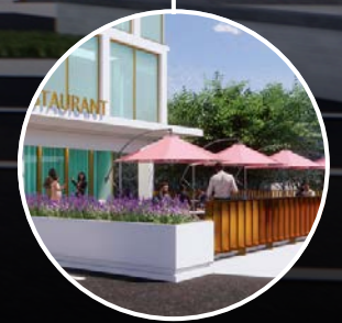
Brand-new patio addition
